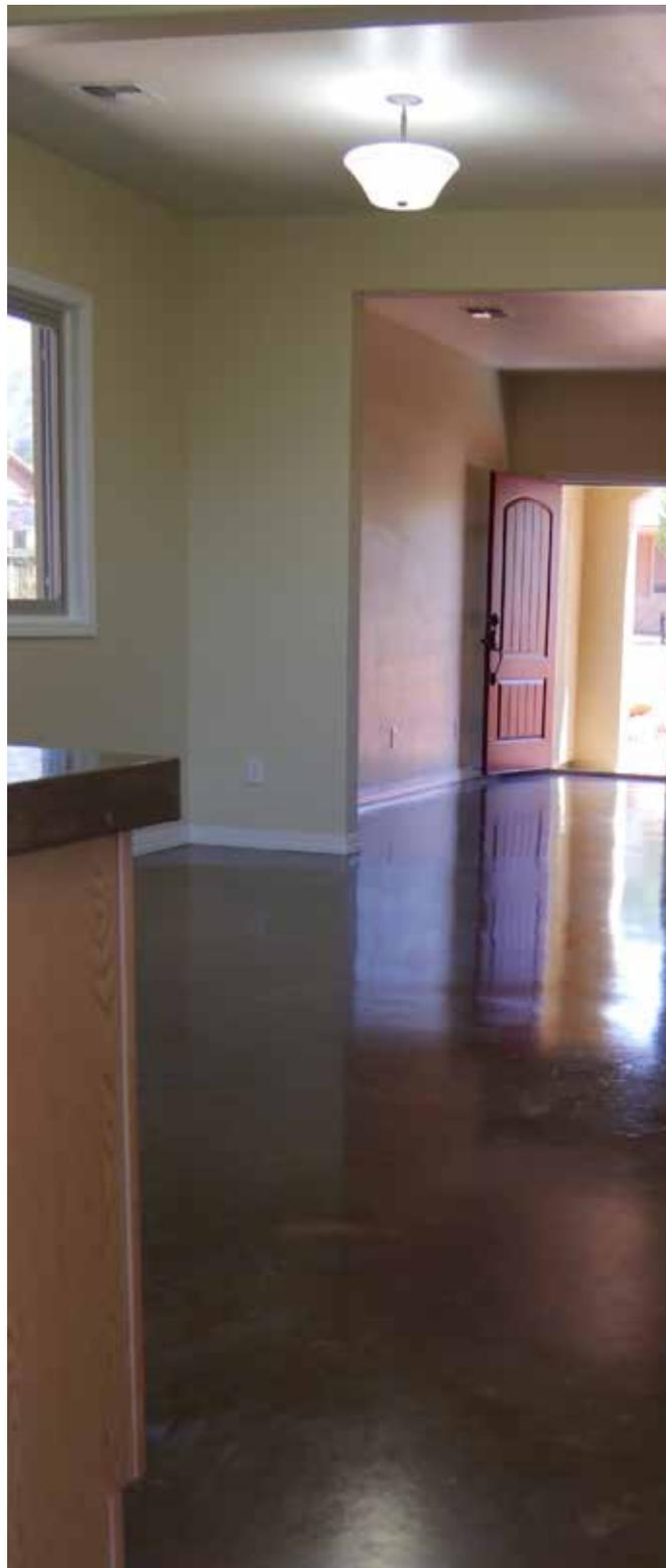
The integrally color concrete floor as acid-stained with Cohill's products: Black Pro Series Chemical Stain and Moccasin Pro Series Earthtone Stain.
